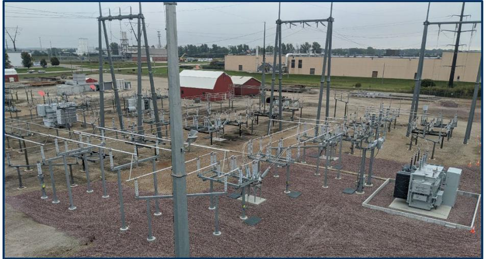
To achieve desired redundancy, OPU tied its new power transformer into SMMPA's 161 kV facilities at the West Owatonna substation. To accommodate the new tie-in, SMMPA converted the 161 kV half-breaker bus configuration into a five-breaker ring bus.
